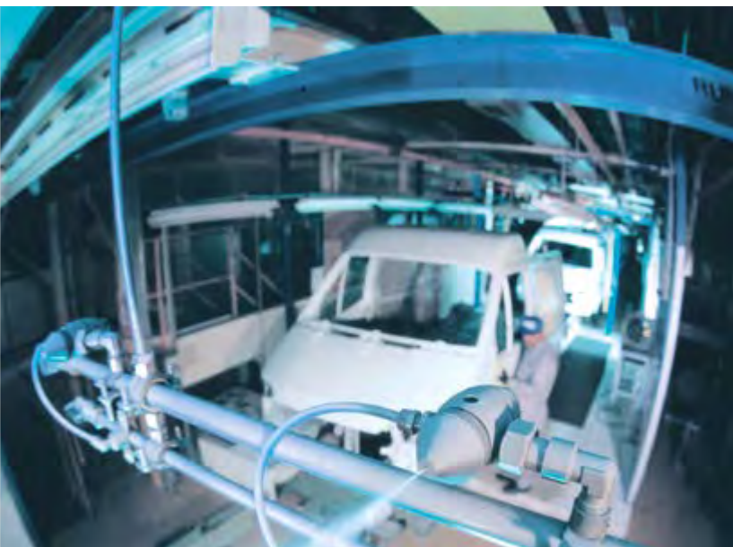
Humidification in an automotive paint shop
