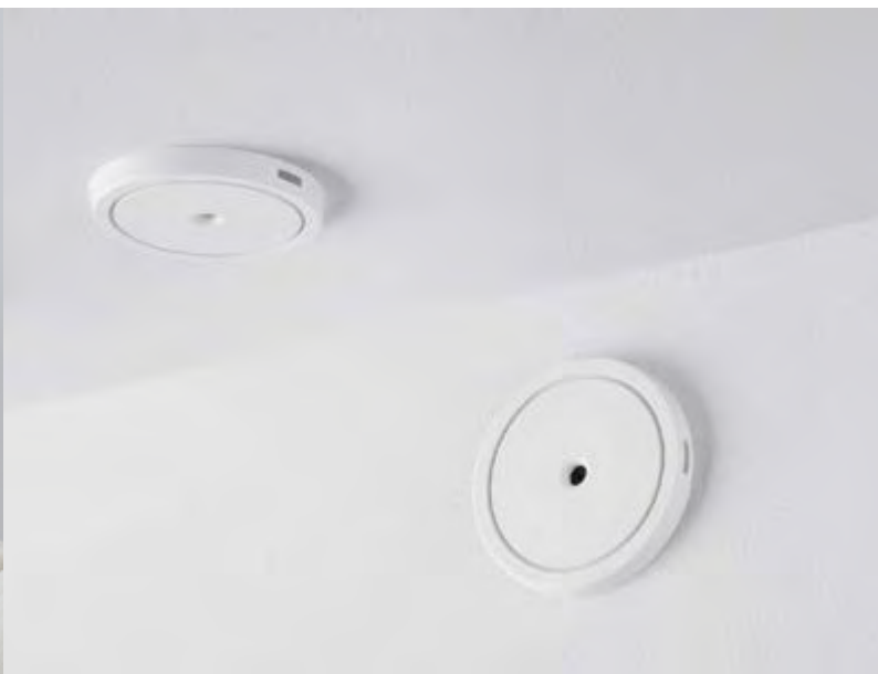
Direct air humidification through humidifier spots
